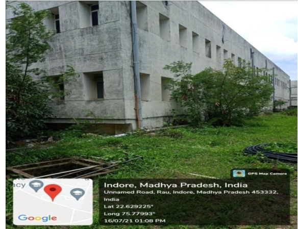
Pit at Back side IIST (C-Block)
