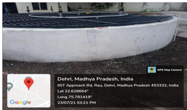
Open well at side of Main Gate
