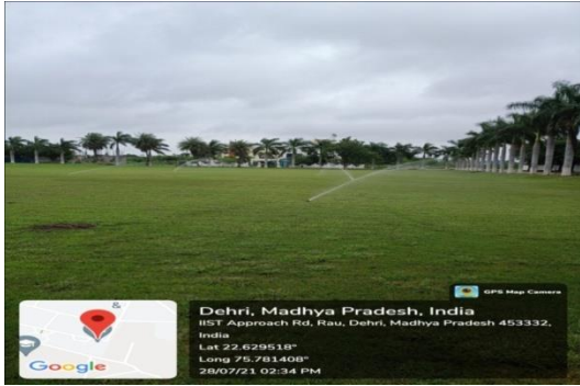
Sprinkler System for watering
