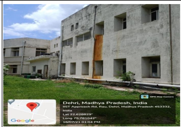
Pipes at Back side IIST (A-Block)
