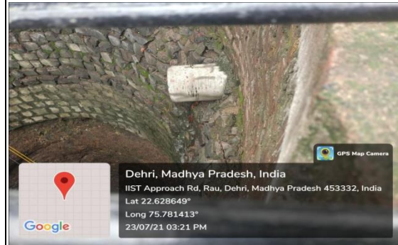
Inlet pipe in well
