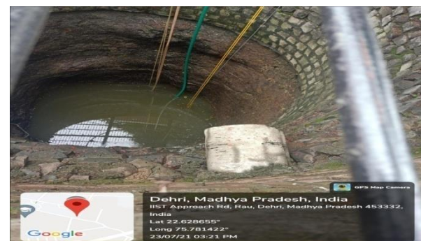
Inlet pipe in well
