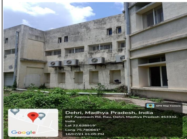
Pipes at Back side IIST (B-Block)
