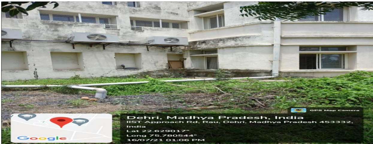
Pit at Back side of IIST (B-Block)
