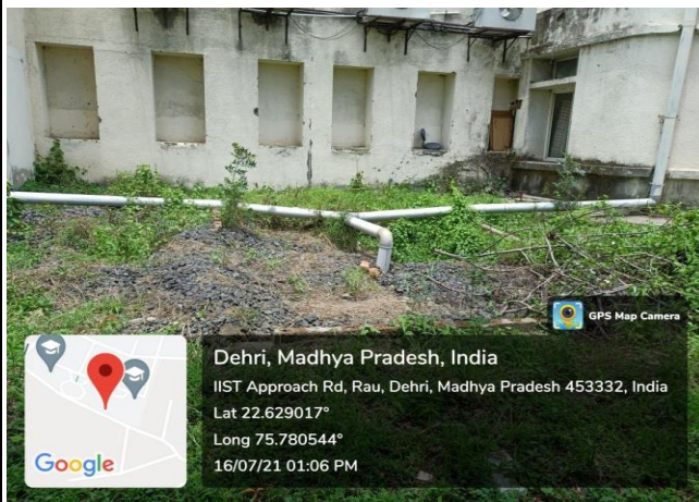
Pit at Back side of IIST (B-Block)
