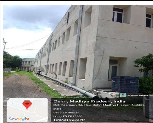
Full view of Pipe line A-C block
