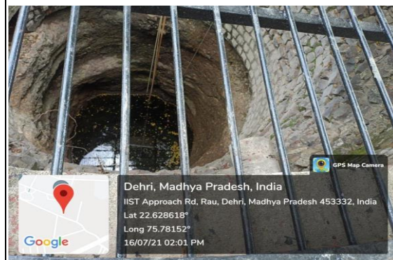
Top view of open well
